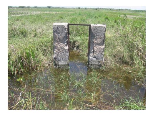
Plate 6: Silted and damaged irrigation canal.
