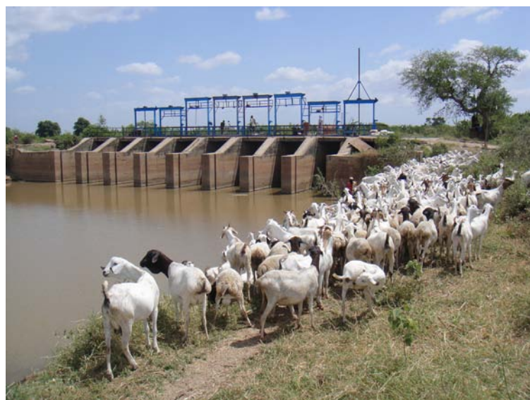
Kurtunwaarey barrage after SWALIM rehabilitation in 2009
