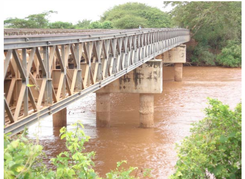
The Marerey bridge
