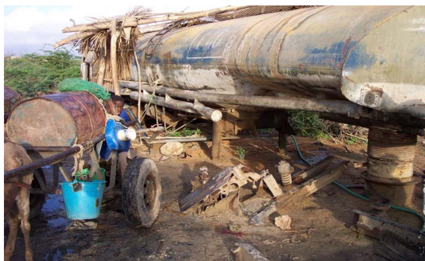
An old oil tank used as water storage tank from a shallow well
