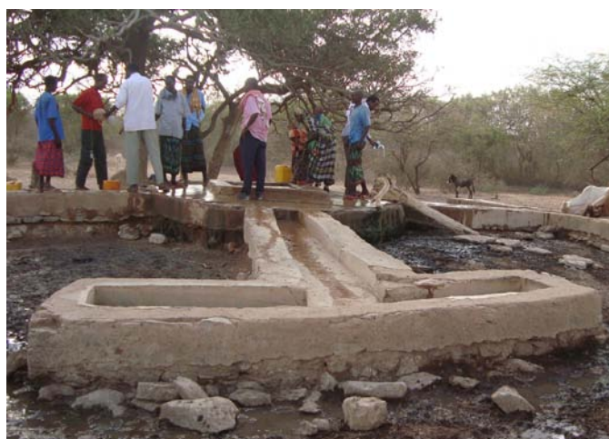
Animal trough connected to a shallow well near Afgooye town
