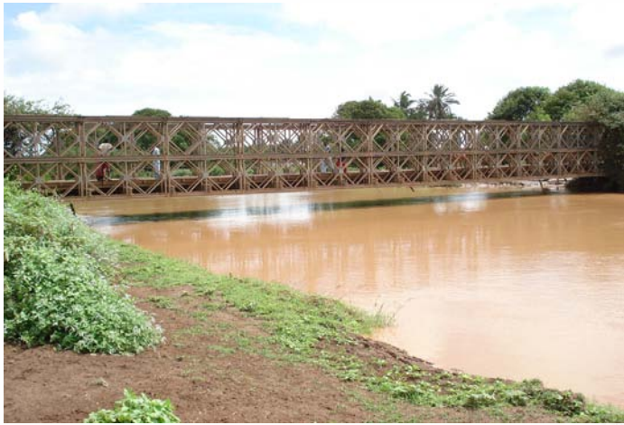
The intense rail network of the Aw Dheegle bridge protects users from falling into the swollen river
