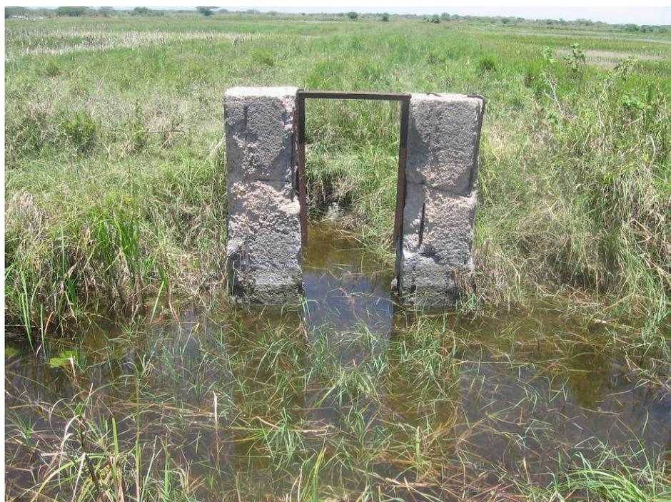
**Plate 6:** Silted and damaged irrigation canal.
