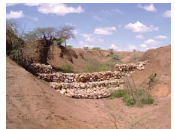
Plate 1 (left) depicts a badland while plate 2 (right) depicts a gully control measure (check dam implemented by IFAD)
